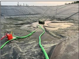
Photo of the drinking water reservoir after it was drained, before the cyanobacteria residue was cleaned. Draining and cleaning of the reservoir took 3 weeks, during which time residents in Sambaa K'e did not have access to treated water. All water tanks in the community were also emptied and cleaned. Photo taken by Rebecca Gasman, York University.
