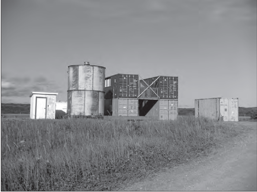
Figure 6. The Bristol Bay Economic Development Corporation constructed this ice machine out of cargo containers to provide fresh ice to fishermen at fish camp in Ekuk, Alaska. The ice keeps the fishermen's catch fresh, which in turn nets a higher profit when the fish are sold to the cannery. Photo courtesy of the author.
