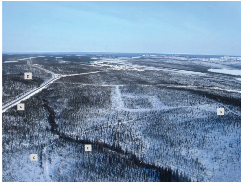
Fig. 1. A variety of linear developments common in northern regions; (A) an all-season road, (B) a snow road, (C) a winter trail, and (D) a seismic line. These types of linear developments often cross watercourses, such as the creek (E), and could impact fish and fish habitat if not constructed and maintained properly. The Inuvik Airport is shown in the background, near the Town of Inuvik, NWT, Canada. Photo: J. Kanigan, GNWT-ENR(CIMP).
