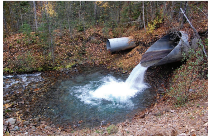
Fig. 3. (A) A perched culvert like this would prevent upstream movement of most species of fish. Photo: K. Maier, GRRB. (B) A decommissioned sump adjacent to a lake in the Mackenzie Delta, NWT. Note the ponding and slumping on top of and around the sump, the different vegetative cover compared to the adjacent landscape, and the drainage towards the lake. Photo: J. Kanigan, GNWT-ENR(CIMP).
