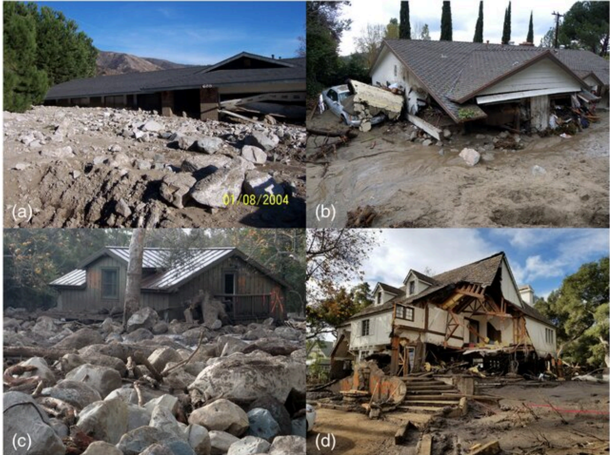
Figure 4: Photos of damage from major postfire debris flows during the last two decades in southern California: (a) December 25, 2003, Devore, San Bernardino County (Old/Grand Prix fires); (b) February 6, 2010, La Cañada-Flintridge, Los Angeles County (2009 Station fire); (c) and (d) January 9, 2018, Montecito, Santa Barbara County (2017 Thomas fire). Photo credits: USGS.
